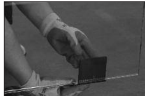
6" (152 mm) edge distance is recommended for most standard applications.
