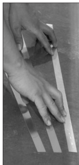
Slide Shim Strips under Base Shoe to fill gaps.
